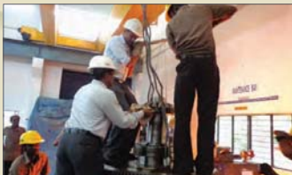
New thrust bearing replacement for U#1 Gearbox
