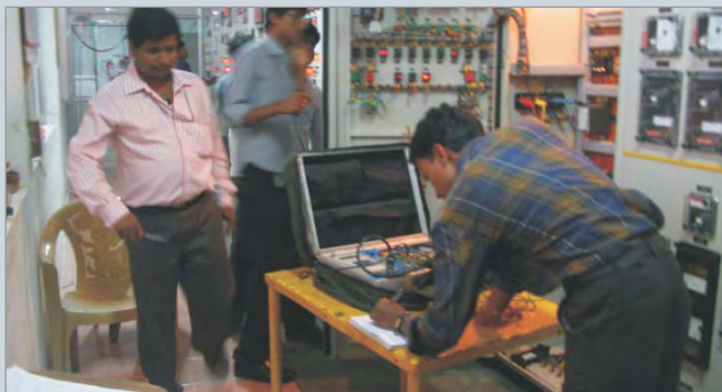
▲ Calibration of the energy meter under progress
