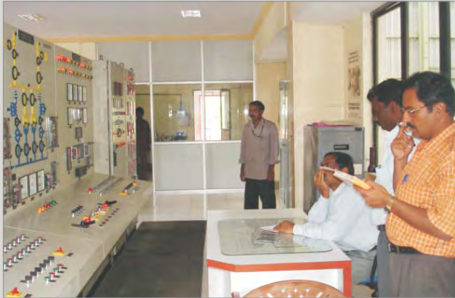
▲ Deputy Chief Electrical Inspector during his visit to the site
