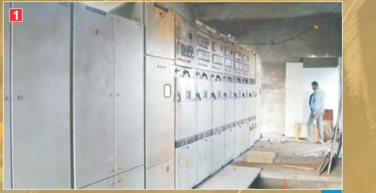
1 Electrical panel has been installed in the switch gear room
