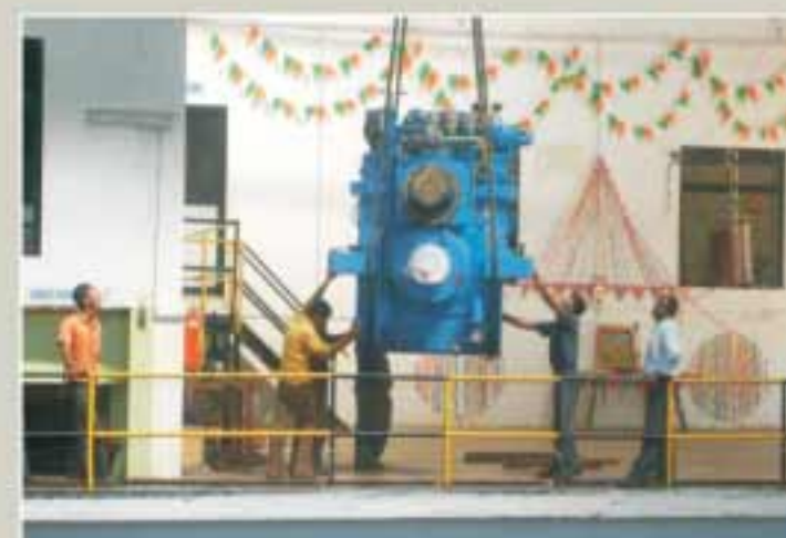
▲ Annual maintenance work under progress
