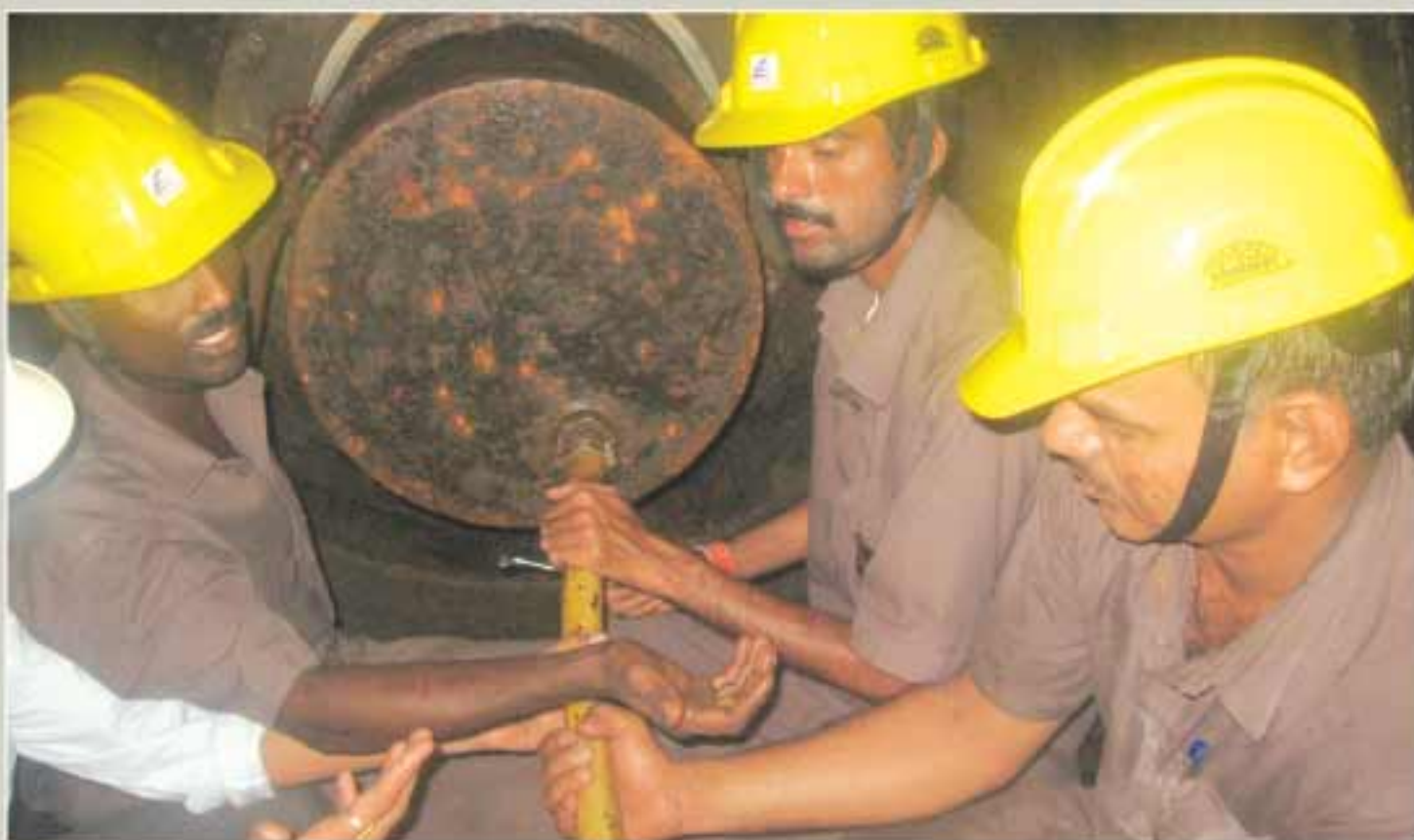
▲ Annual maintenance work under progress
